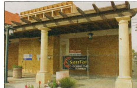
BREWING: San Tan Brewing Company is under construction in downtown Chandler.
